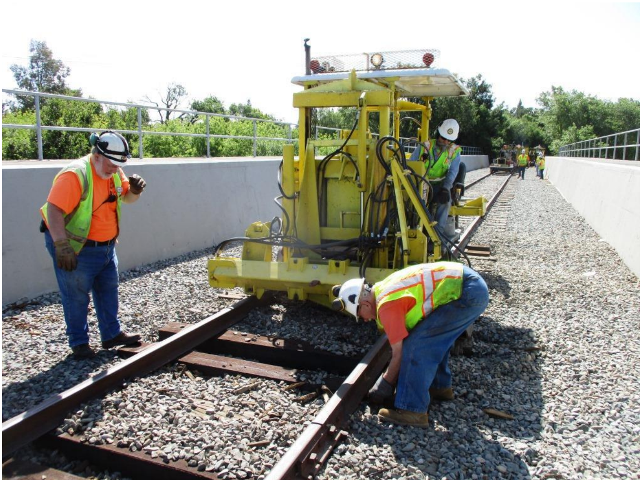
Joe uses the 125's track-jacks to lift the rail slightly for Frank and Clem to insert tie-plates
