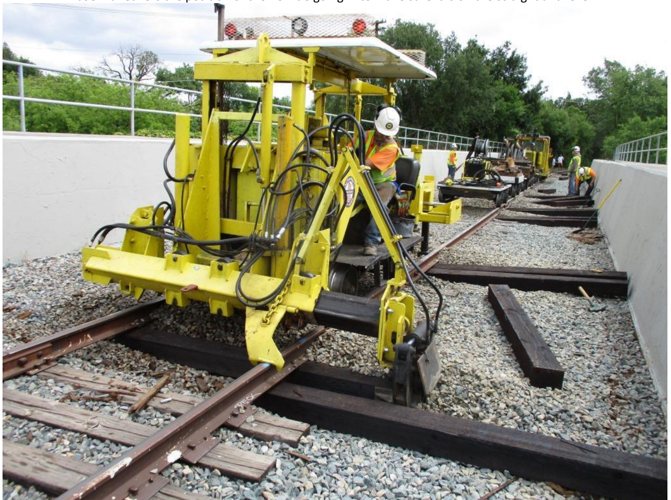
Joe used the inserting ram to move ballast about in order to provide a level surface
