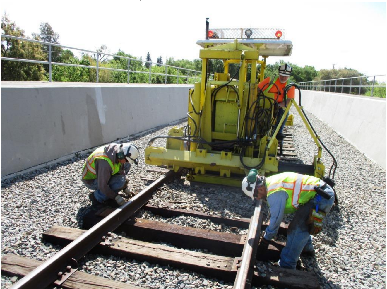
Frank takes a turn on the 125 as Steve and Joe insert tie-plates
