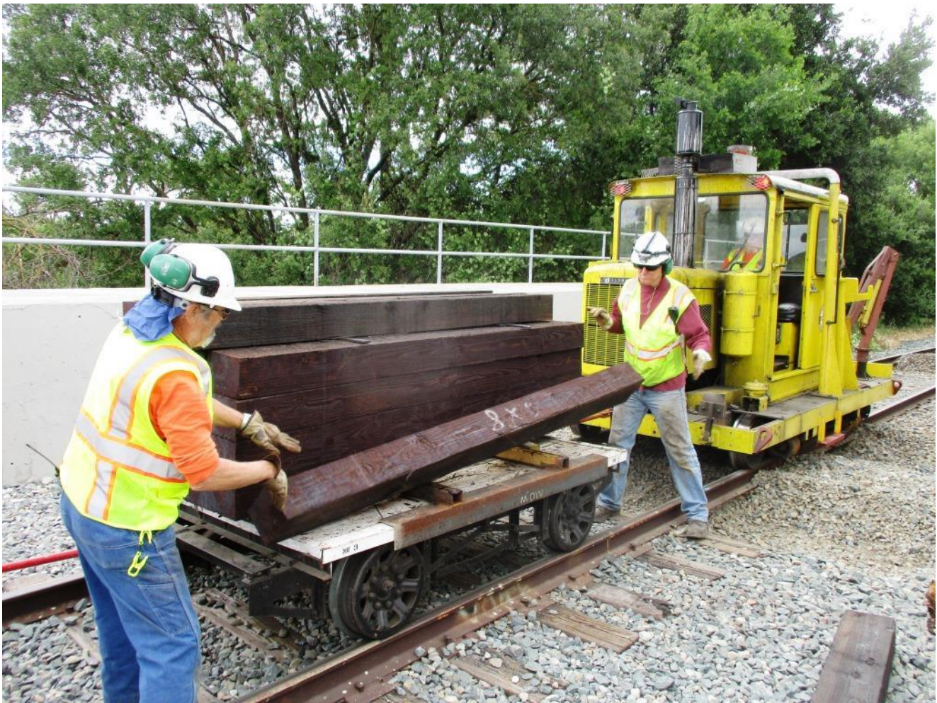
Ties fly off o the pile as Ed and Steve drop new ties next to the now empty tie-cribs
