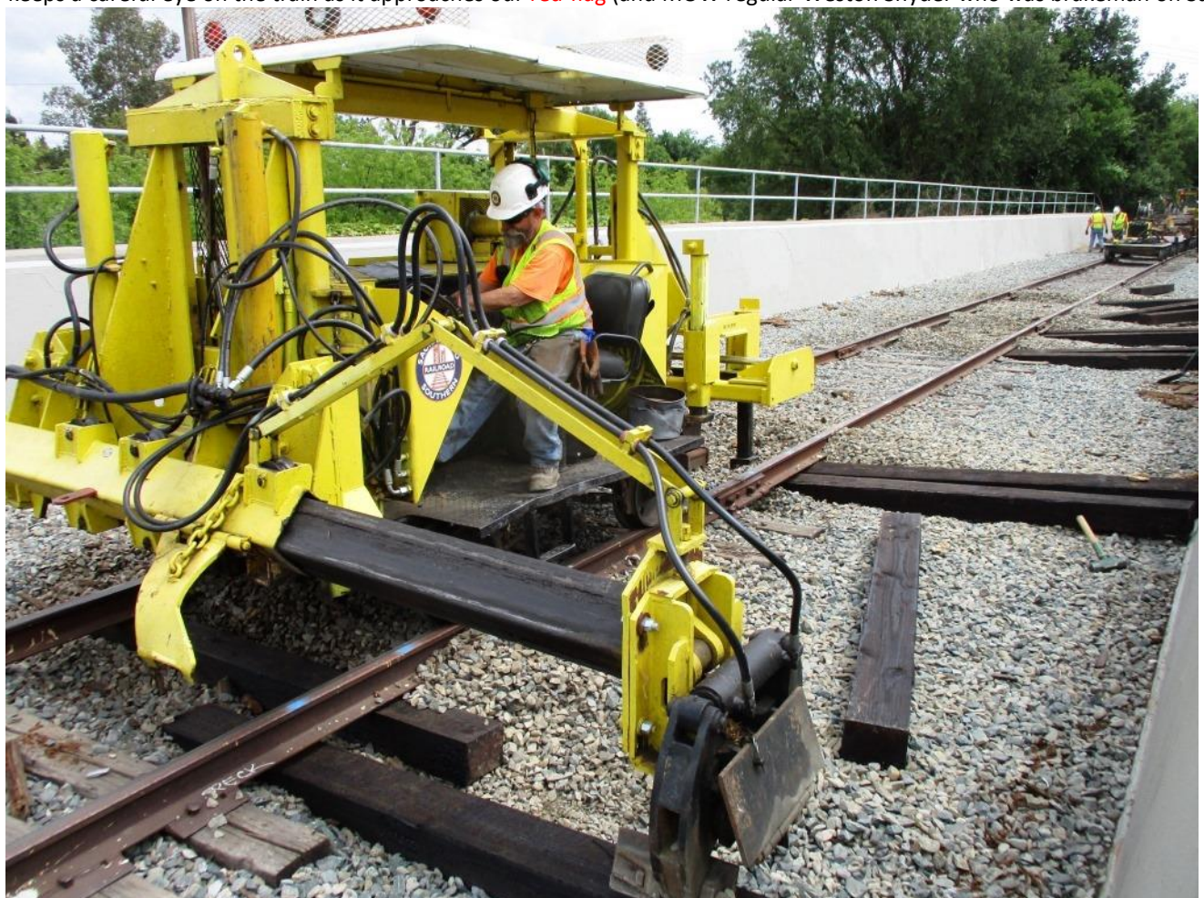
Joe manipulates the insertion ram on the 125 to prevent the ties from “submarining” as the wall forces them to be placed at an angle
