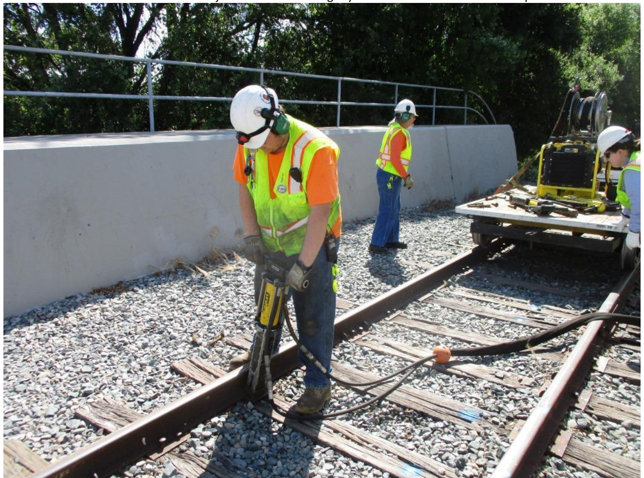
Chris deploys the hydraulic spike puller
