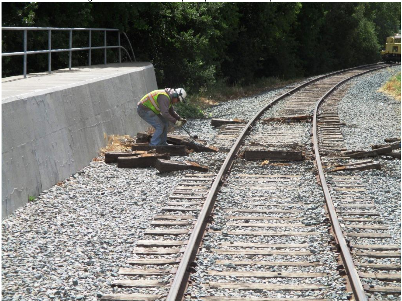
In its wake, the tie-shear leaves nothing but splintered debris which Steve clears away from the track
