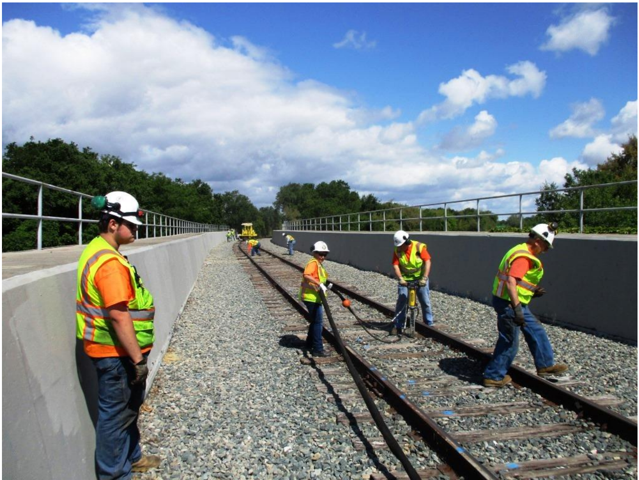
From one end of the bridge to the other, the MOW Team works on bringing the track up to federal Class 2 standards
