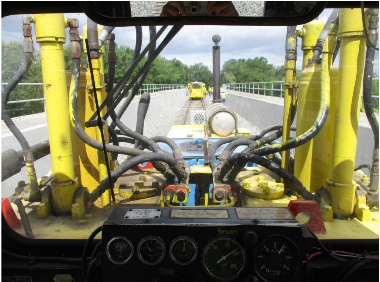
Bring in the tie-shear! With spikes pulled, the tie-shear now slices its way through the nasty old ties
