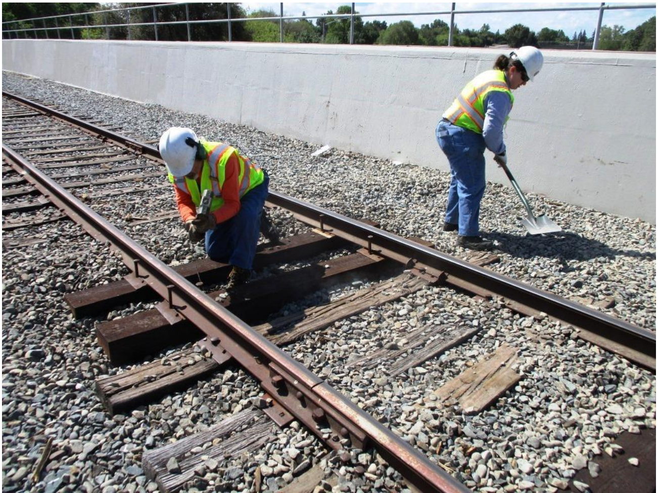
Ed sets spikes as Heather fills in holes in the ballast
