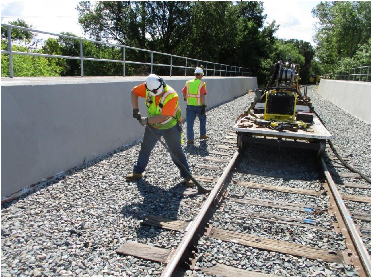
For spikes that were too close to joint bolts for the hydraulic puller to grab, Chris uses the tried and true method of removing them
