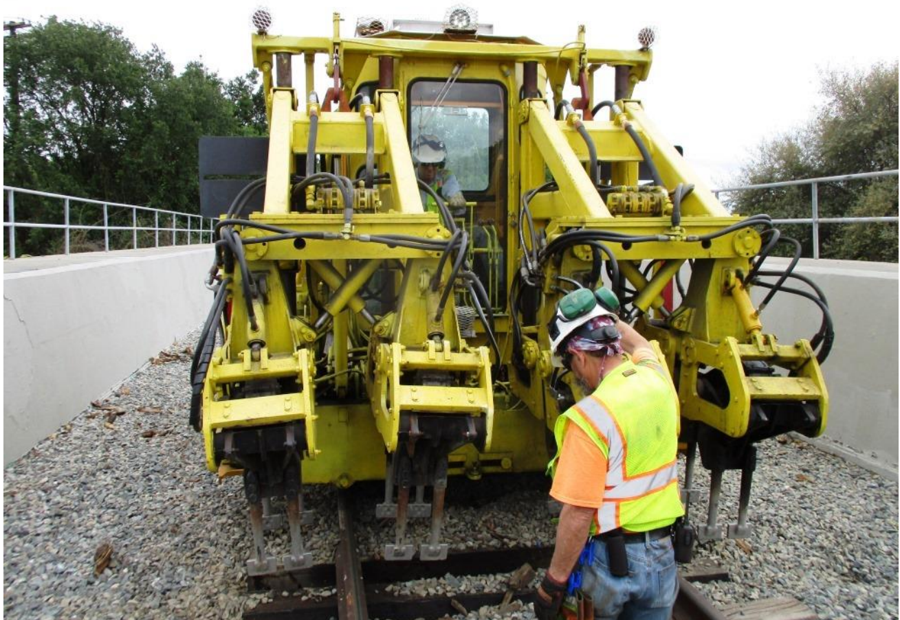
With all the ties inserted, Steve brings the tamper in to tamp the ties flush with the rails
