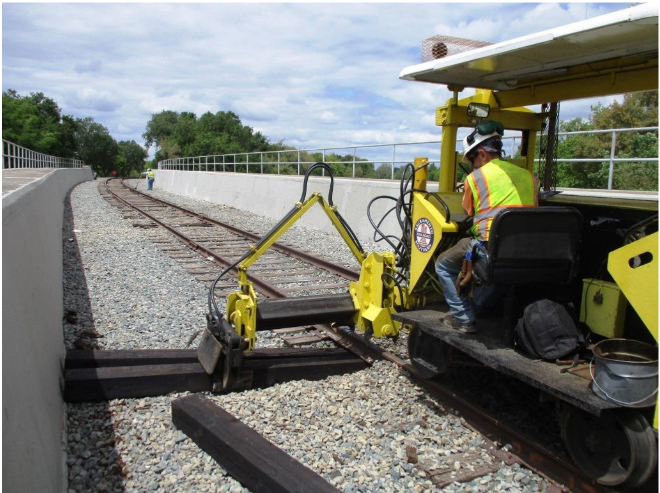
Joe maneuvers the position of the new tie going in to make sure it is on the straight and level
