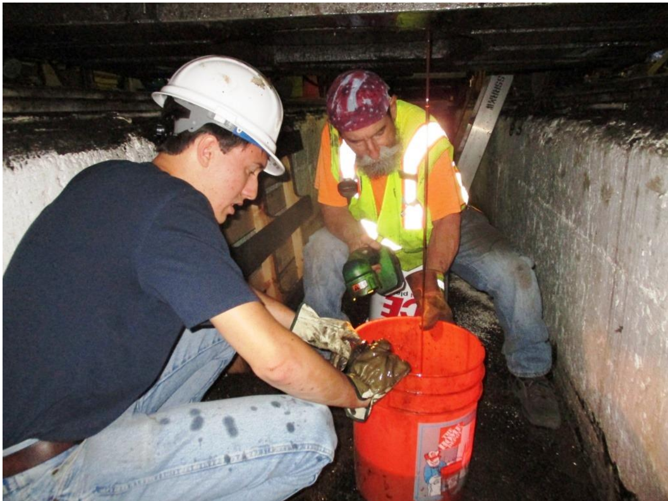
In the “pit of despair” under the Kalamazoo, Jack and Joe drain the sludge from the transmission (drenching Jack in the process)
